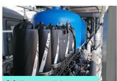
Ref.: Pharmaceutical industry APPLICATION: Multimedia filter protection in a sea water desalination plant FLOW FLOW: 120 m<sup>3</sup>/h LOCATION: Spain
