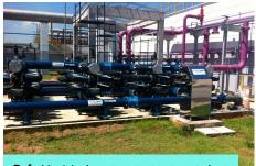
Ref.: Municipal wastewater treatment plant APPLICATION: Protection of microfiltration cartridges FLOW: 500 m<sup>3</sup>/h LOCATION: Brazil
